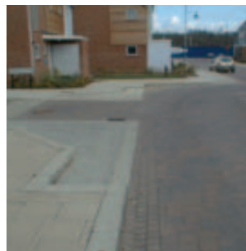
A gentle ramp and change in surface material slows vehicles at junctions whilst allowing larger vehicles to manoeuvre. (St Mary's Island, Ventura)
